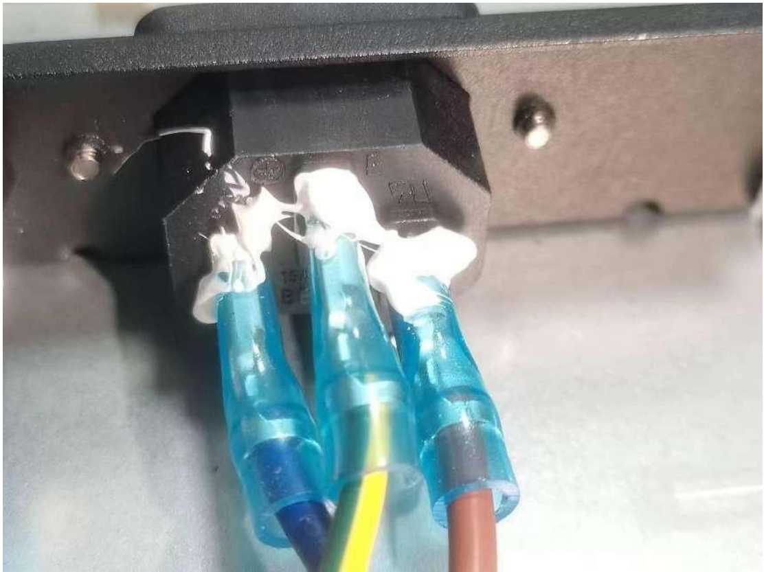
Figure 16. Earthing terminal view
